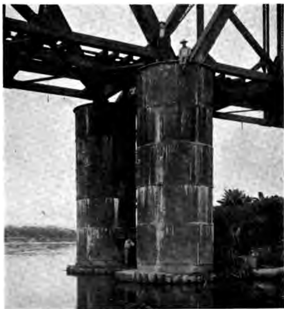
Steel Sheet Piling
